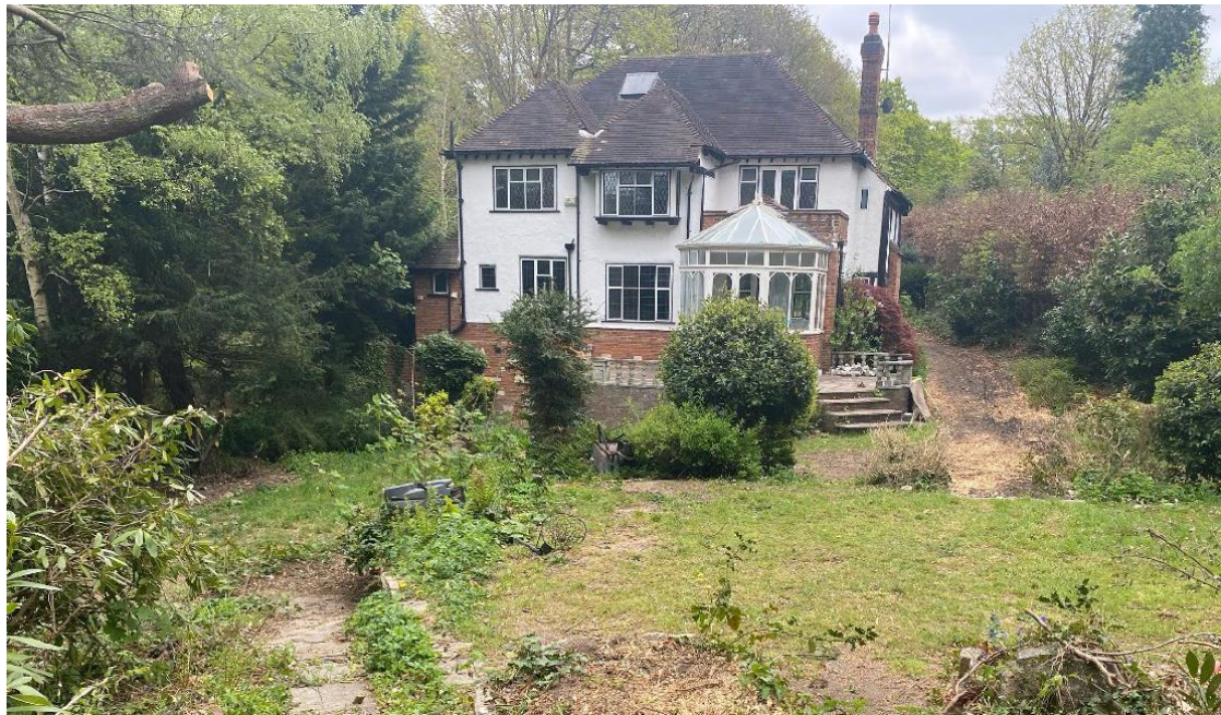
Figure 4: Rear of existing dwelling
